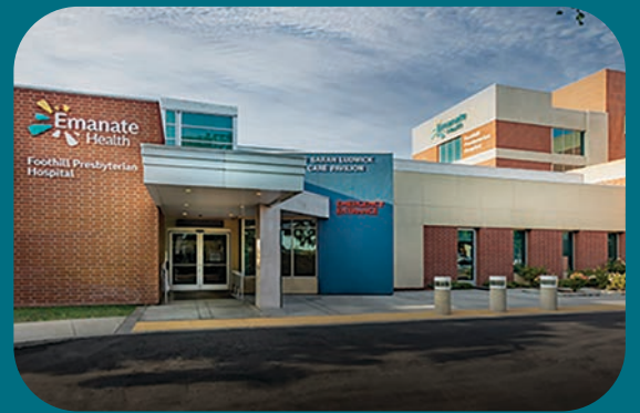
Foothill Presbyterian Hospital
