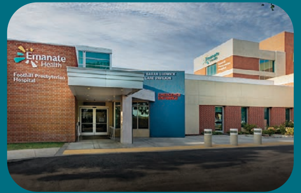
Foothill Presbyterian Hospital
