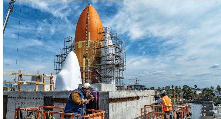
of moving, lifting, and stacking each shuttle component into its vertical configuration. "Go For Stack" began with installing the 13,000-pound aft skirts, which serve as Endeavour's foundation, attaching and securing the shuttle to seismic isolators beneath the building. The seismic isolator pad is built to bear the weight of the 500,000-pound shuttle, measuring about eight feet thick, 45 feet wide, and 75 feet long.
